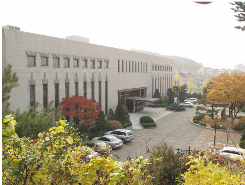
The NAS Building
